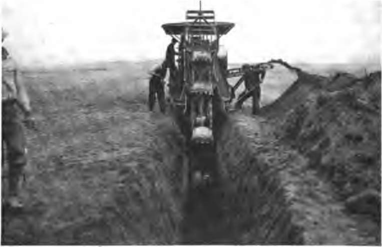
FIG. 61.—Excavating Trench for Tile Drain, Montana.
